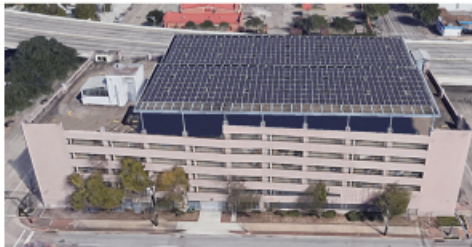
Figure1. Photovoltaic System at the Site
